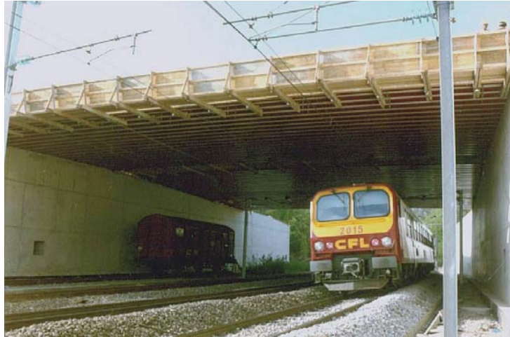
Fig. 7: Highway bridge in Luxembourg with a slenderness of 42
