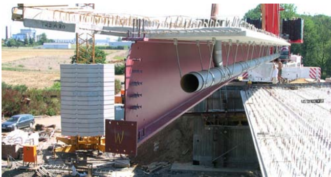
Fig. 5: Placing of the prefabricated composite beams
