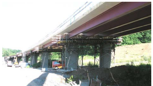
Fig. 6: Almost finished Horlofftal bridge
