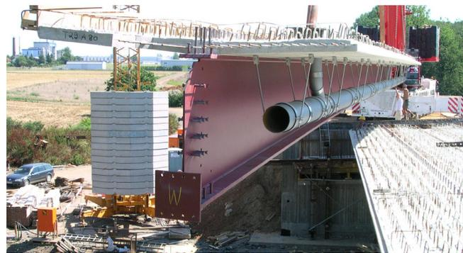
Fig. 2 – VFT®-solution with rolled steel beam
