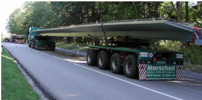
Fig. 6 – Transport of the VFT-WIB girders from the concrete plant to the construction site
