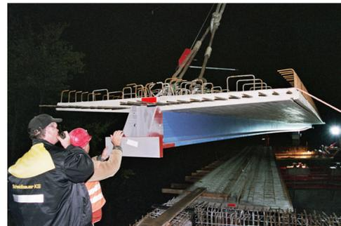
Fig. 7 – Placing of the VFT-WIB girder with 32.50 [m] length
