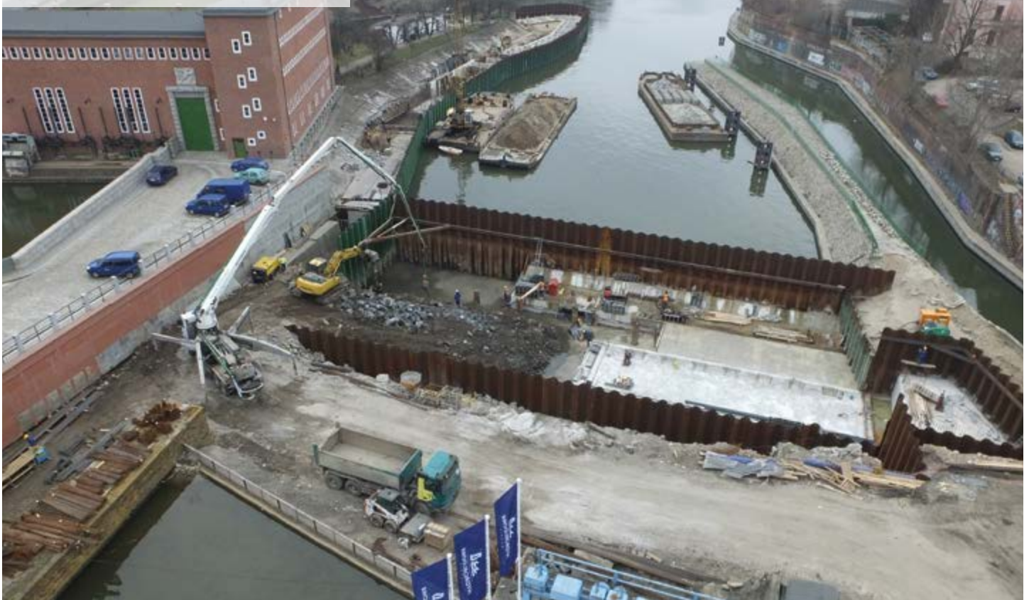
Wroclaw flood protection system, Poland
