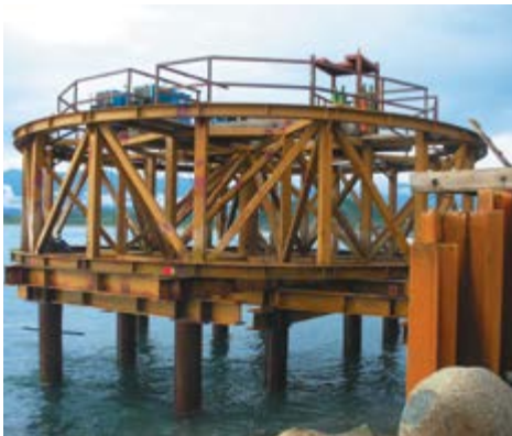
1. Installation of template
