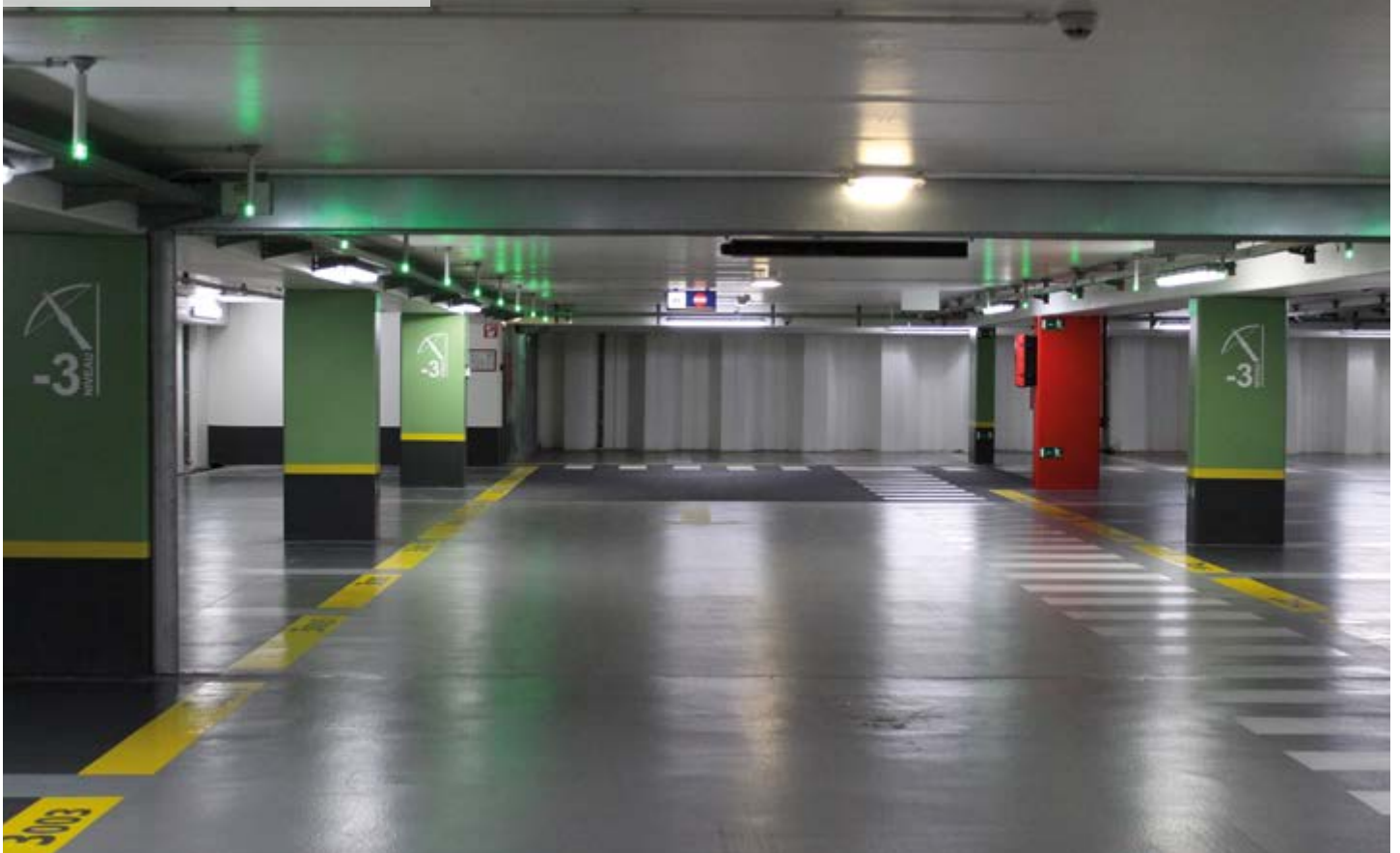
Underground car park, Aalst, Belgium
