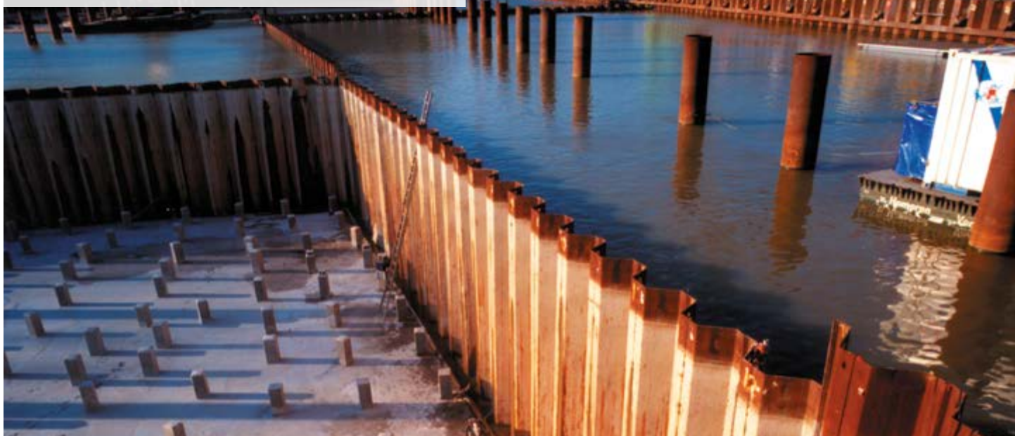
Excavation for an office building, Amsterdam, Netherlands
