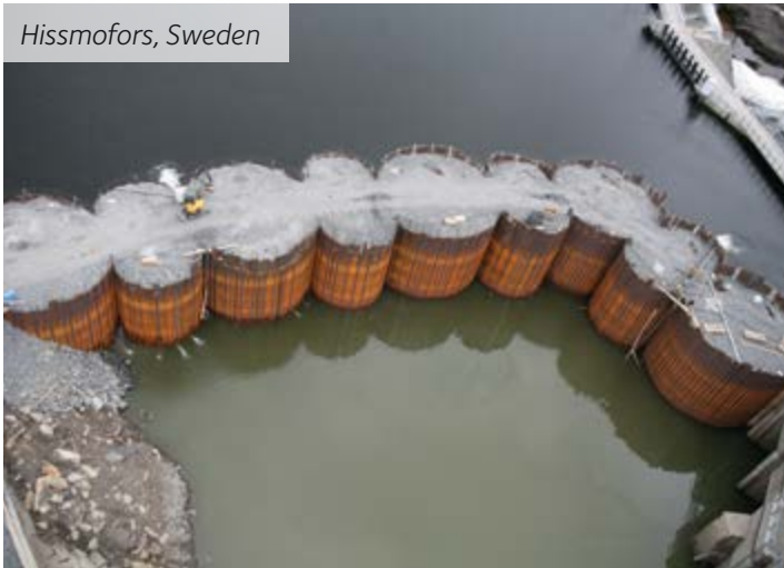
Circular cells with 35^\circ junction piles and one or two connecting arcs.
