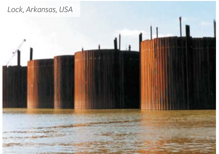
Diaphragm cells with 120^\circ junction piles.
