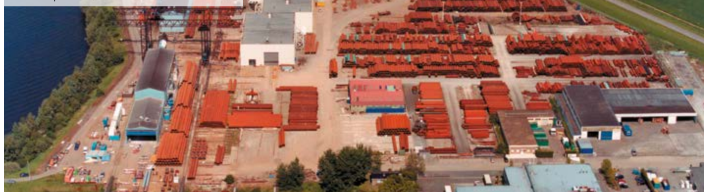
Tubular pile mill, Dintelmond, Netherlands
