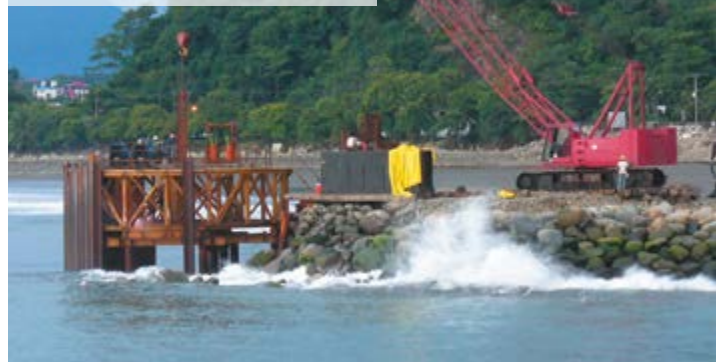
Marina breakwater, Costa Rica
