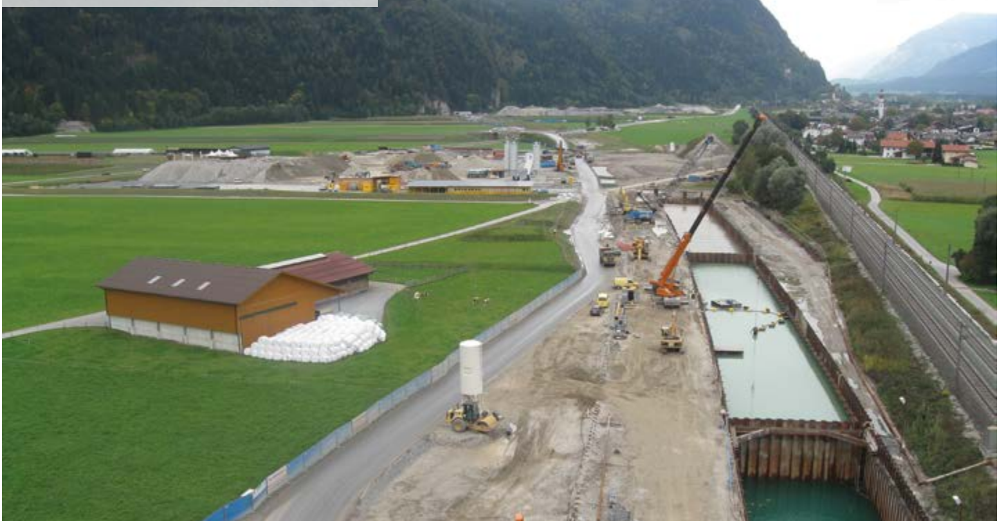
Temporary trench, Brenner motorway Austria
