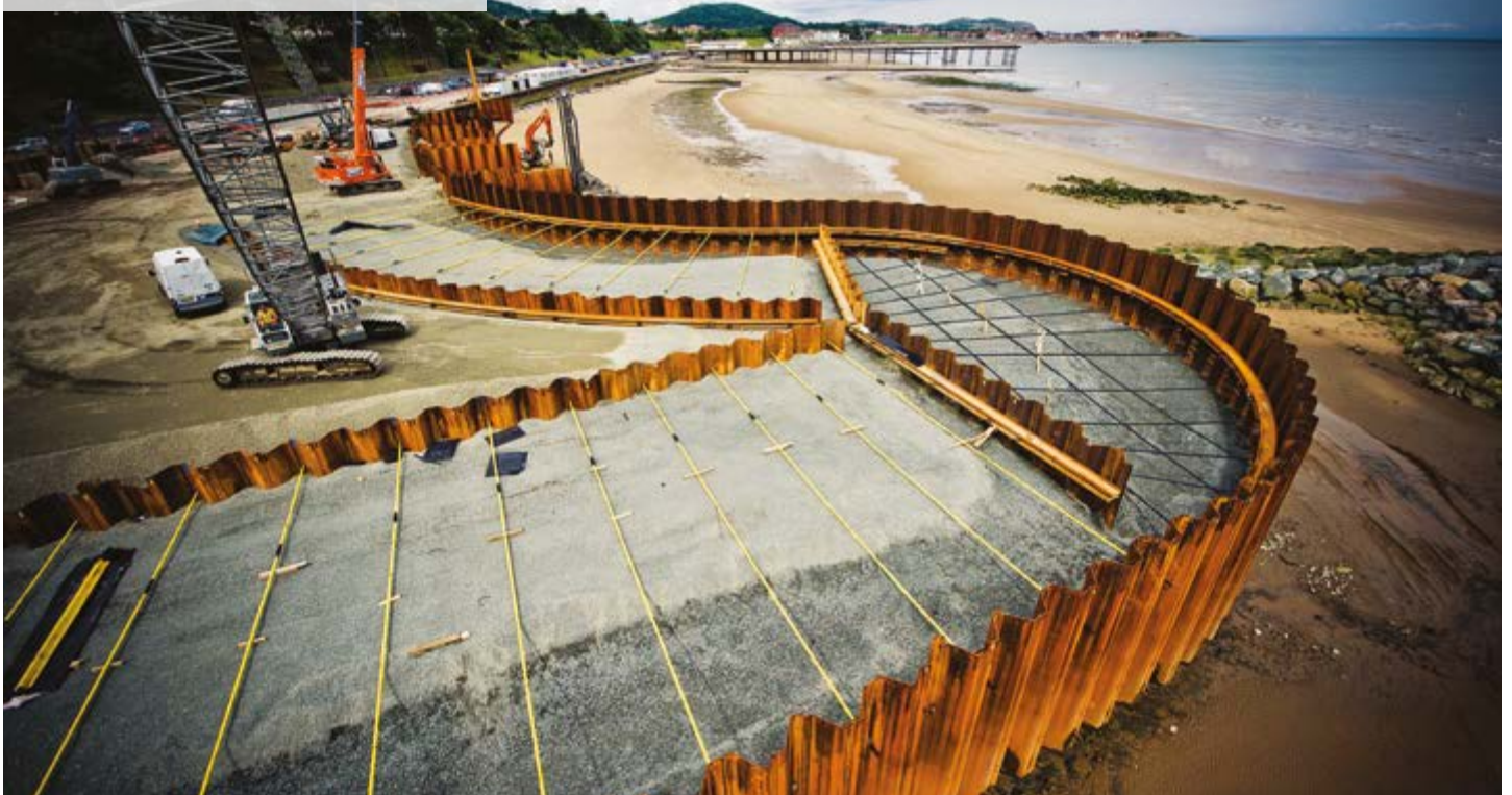
Costal defense project, Colwyn Bay, UK
