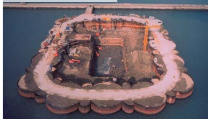
Bridge construction, South Korea
