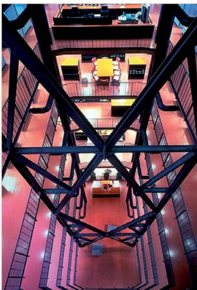
ArcelorMittal office building (AOB), Luxembourg
