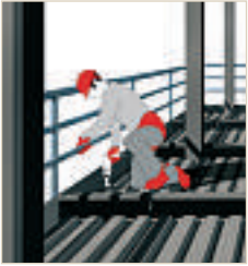
Fixing and stitching of the floor deck
