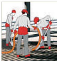
Pouring of concrete
