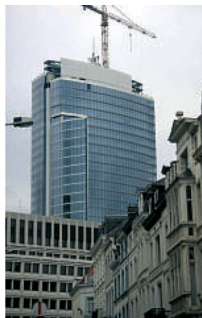
Tour Madou, Brussels (Belgium) ARCHITECTS: Assar/archi 2000
