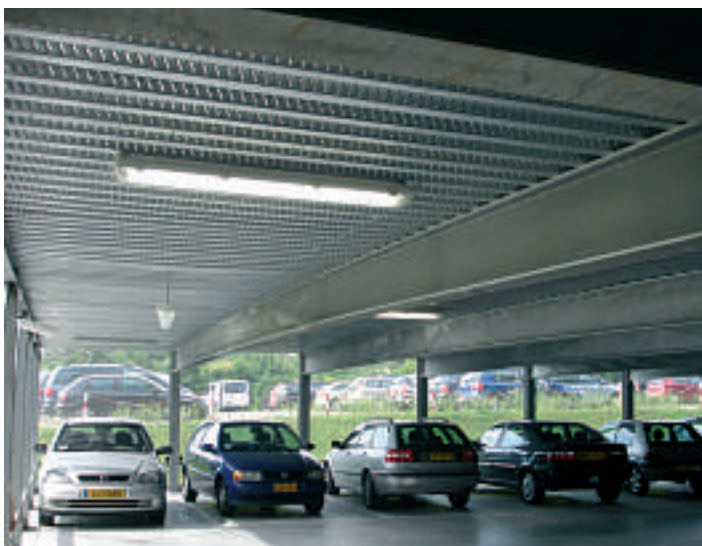
Photo on top: Car park Carrefour, Aix-les-Milles (France) ARCHITECTS: Sud architectes (Y. Melia)
