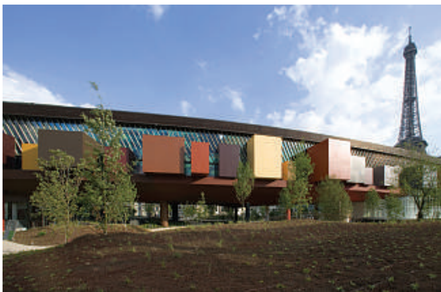
Quai Branly Museum, Paris (France) ARCHITECTS : Ateliers Jean Nouvel
