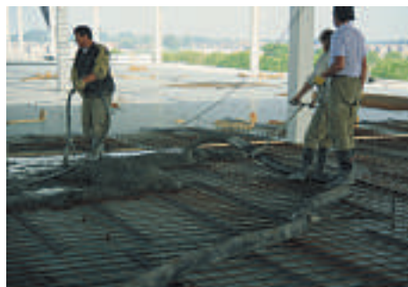
On site concrete pouring of the slab
