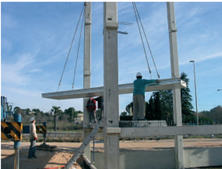
Installation of a prefabricated floor
