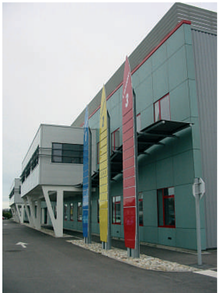
Building E. Placenet, Saint-Martin-Boulogne (France) BET: Maning
