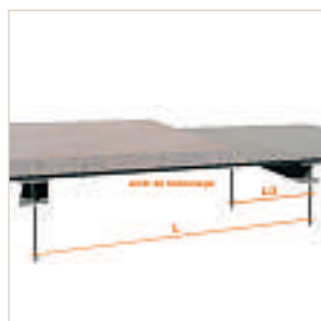
9. Adjust the slab as work progresses
