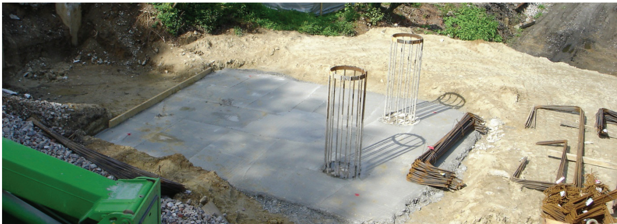
Figure 5-3: Concrete piles used for Entenpfuhler bridge in Germany (connecting reinforcement)
