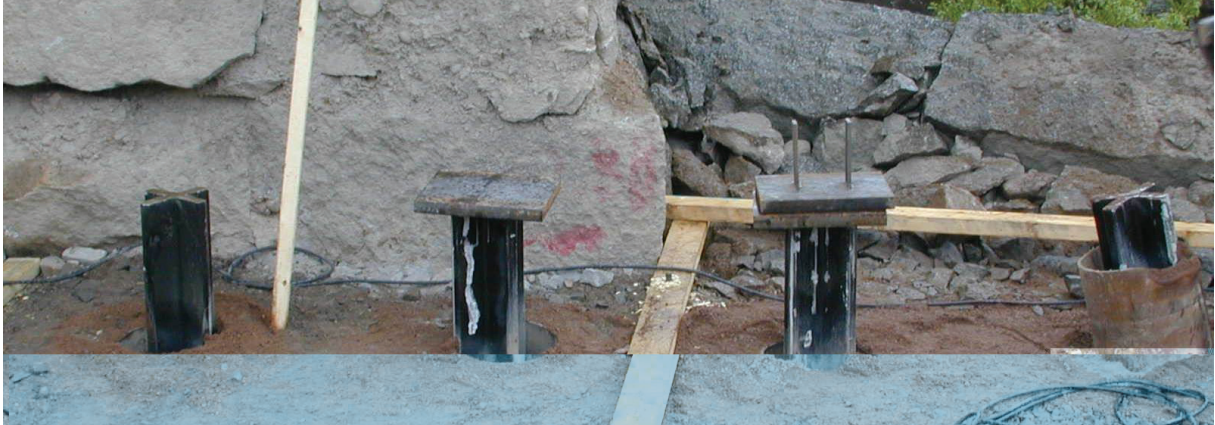
Figure 5-2: X-piles used for Leduån bridge in Sweden, surrounded by loose sand
