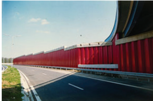
Figure 9-6: Soleuvre bridge, South Motorway, Luxembourg, (conventional bridge) (ArcelorMittal Long Commercial, 2003)
