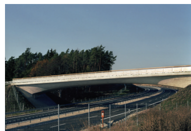
Figure 1-8: Integral abutment bridge with inclined abutments
