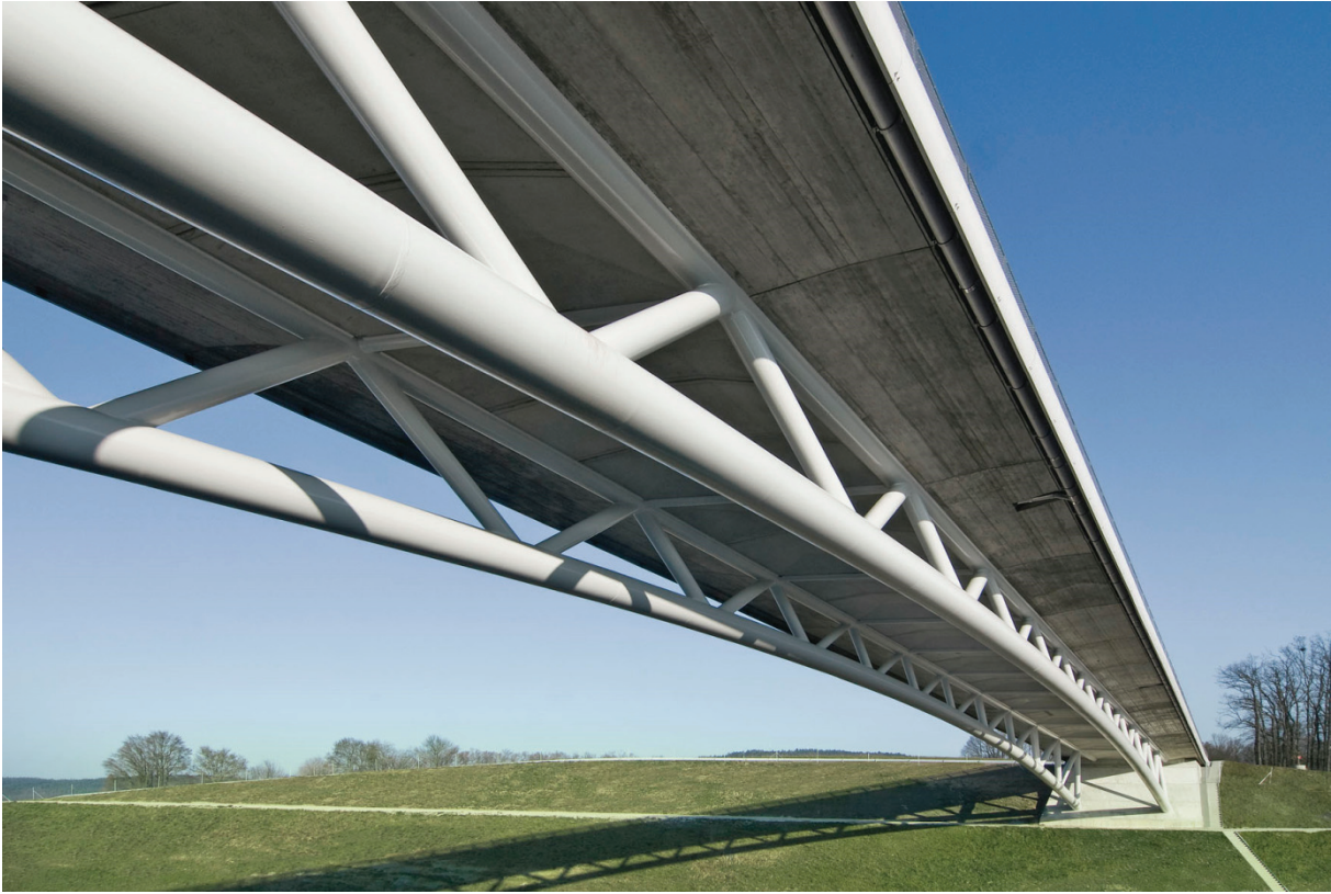
Figure 1-2: Composite bridge with integral abutments by SSF, A73 (Munich), Germany
