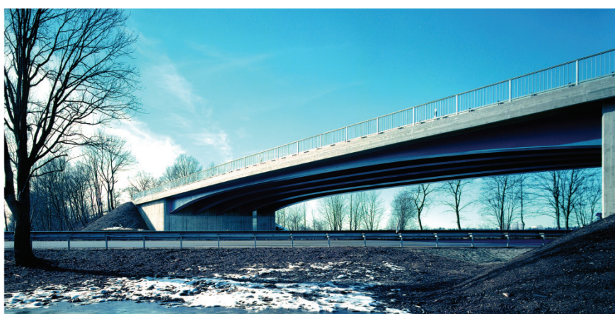
Figure 1-5: BAB A8 bridge structure 5 (SSF), foundation with high flexural stiffness
