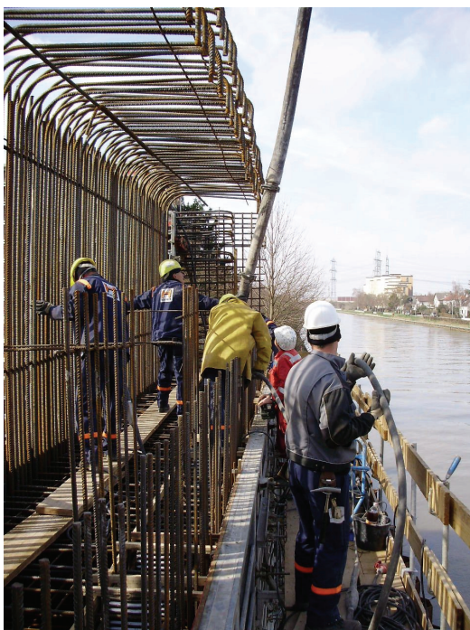
Figure 13-3: placement of reinforcement
