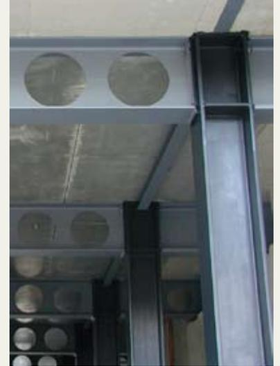
Figure 17 Beam to column connection
